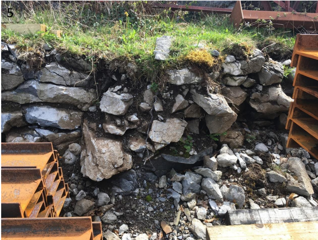
5. Cross section of lands exposed on ledge at eastern boundary of the "new " yard, adjacent to Shed 3, showing fractured bedrock
